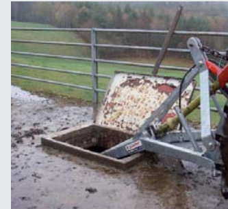
Pit under shed with reduced opening
