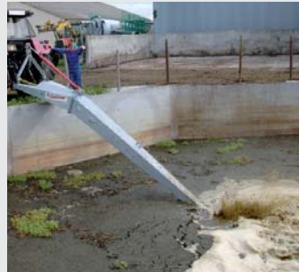
Round or squared concrete pit
